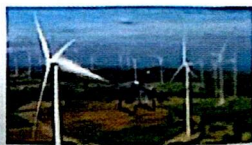
Wind Turbine Maintenance
