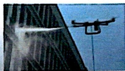
High-Rise Building Cleaning
